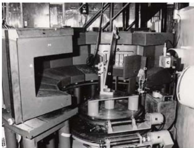
*A specially designed specimen rig in place on the HRPD at HIFAR. Note also the approximately 120 degree detector bank on the HRPD.*
