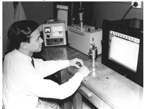
AINSE tritium gas counting equipment in use in 1961, described above
