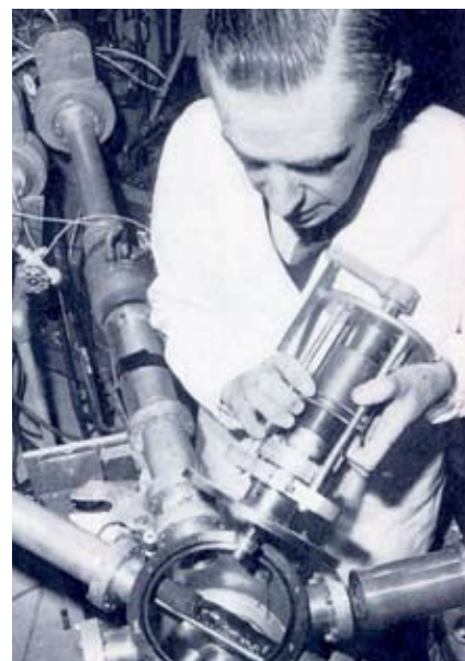
Roger Bird loading obsidian samples into the PIGE analysis chamber on the 3 MV Van de Graaff accelerator in 1975.
